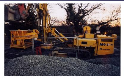
Emergency Infilling of a high risk part of the Daw End Limestone Mines system in Aldridge due to collapse of workings which had closed Bosty Lane and threatened adjacent property. The workings were between 30 – 40m bgl and were flooded.
